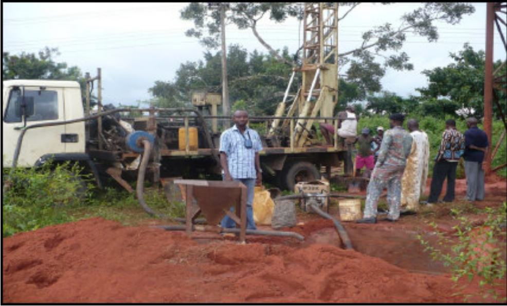
Above: Drilling a deep well at Igueben
